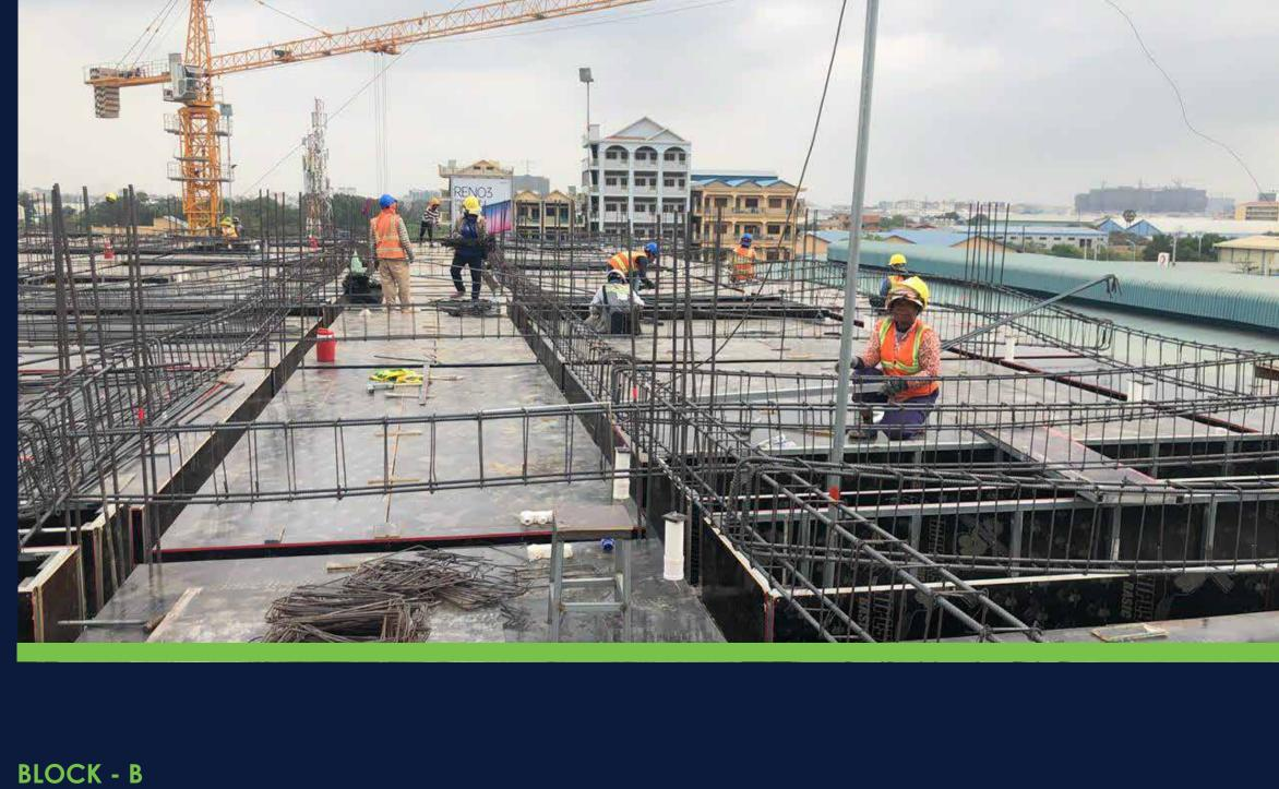
2nd storey slab formwork and rebar installation in progress.
