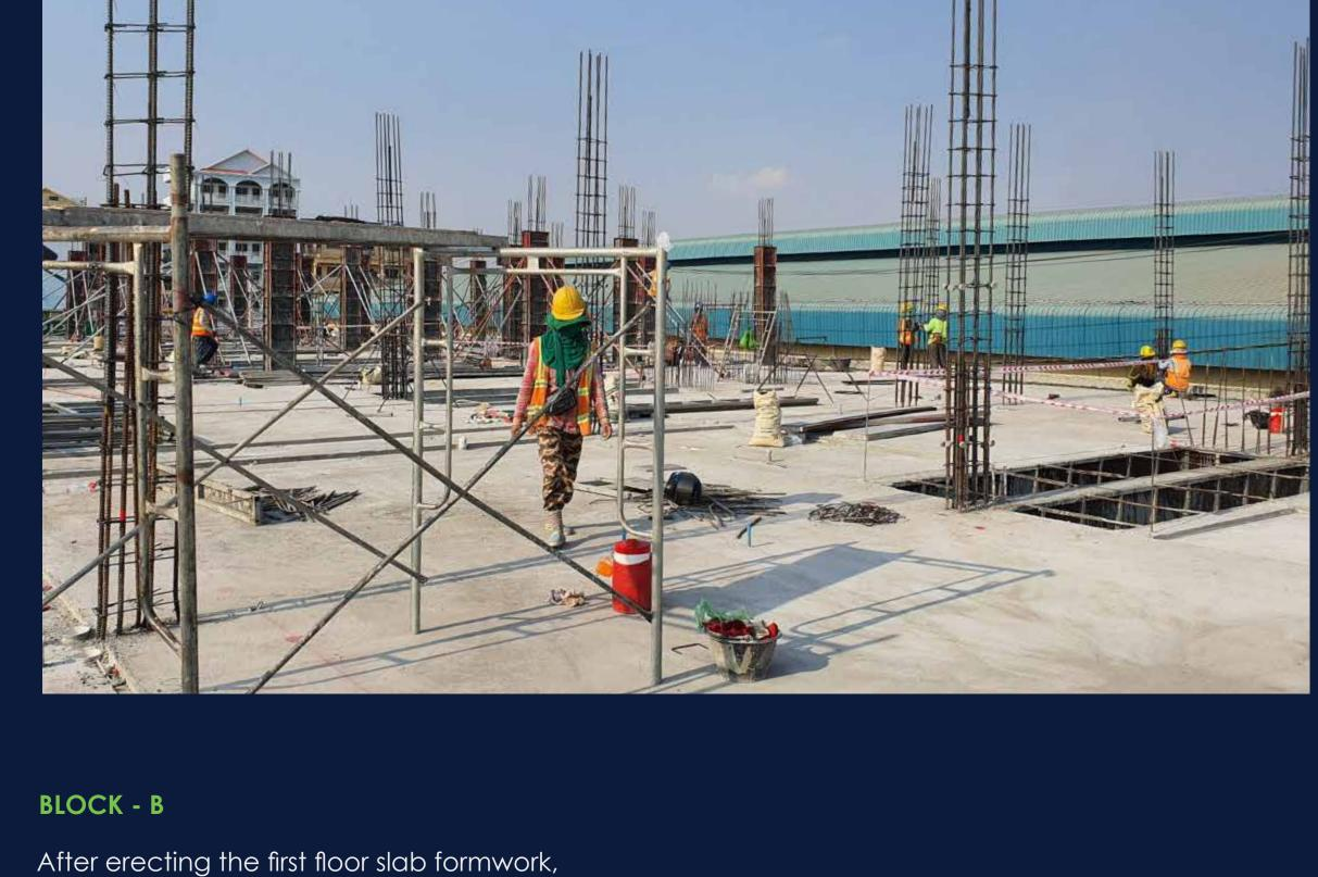
we are now reinforcing the first floor beams and slabs.
